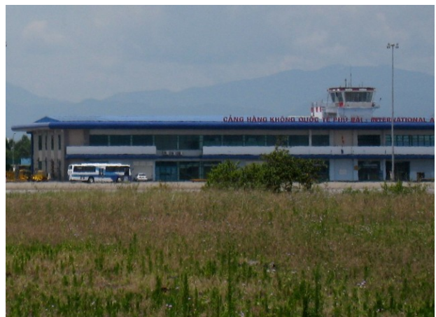
Phu Bai International Airport built around the deactivated tower used by Marines during the Vietnam War. The grassy area in front of the terminal was the VMO-3 operations area in 1967
